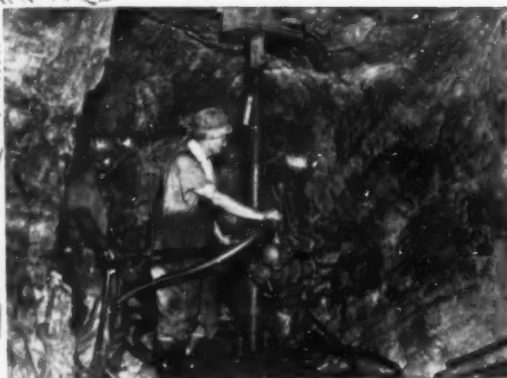
CP-55 drilling in advance of development heading to test for high-pressure water pockets.
